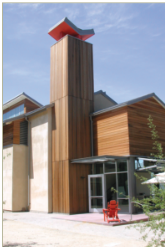
Fig. 4. The new building for the Department of Global Ecology on the Stanford campus was dedicated in April 2004. Its orientation reduces heat buildup, and temperature control is achieved naturally with a cooling tower.
