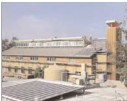
▶ Fig. 2. The new research building for the Department of Global Ecology is scheduled for completion in spring 2004. It was designed with many high-performance features to maximize energy efficiency, minimize waste, and enhance occupant comfort. This photo was taken in January 2004.
