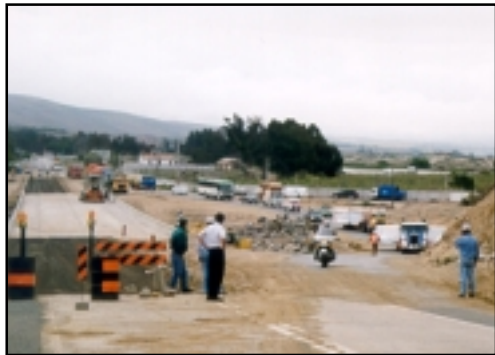
The convoy makes a detour around an almost-completed bridge on the Pan American Highway.
